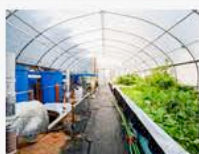
4 Cylburn Aquaponics Project
