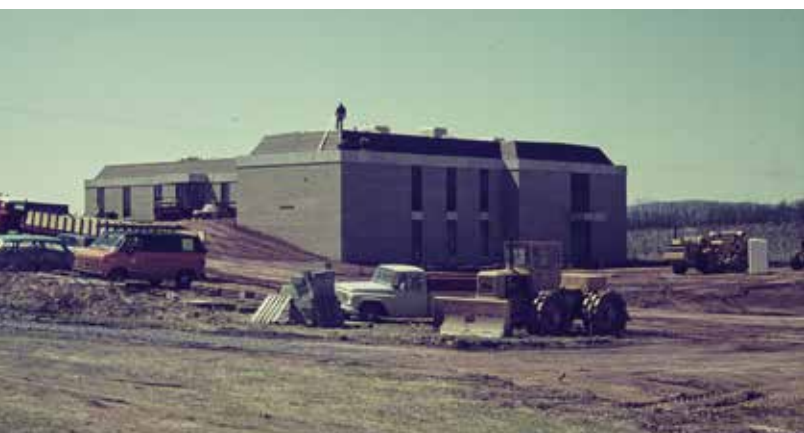
Musselman Building under construction
