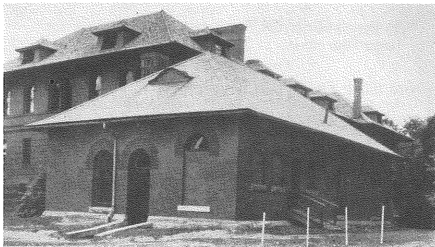
FIG. 1. RESPIRATION CALORIMETER BUILDING, THE PENNSYLVANIA STATE COLLEGE
